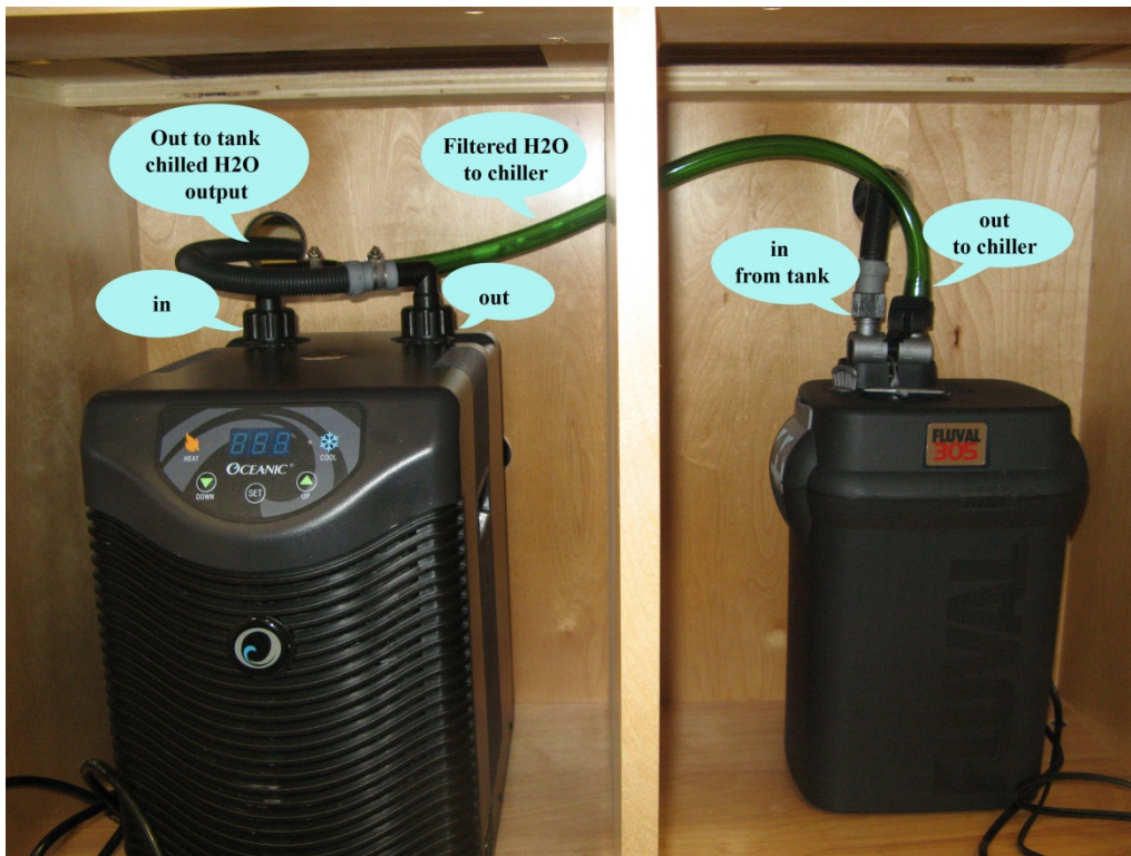
Figure 4 Correct arrangement of tube connections for filter and chiller
